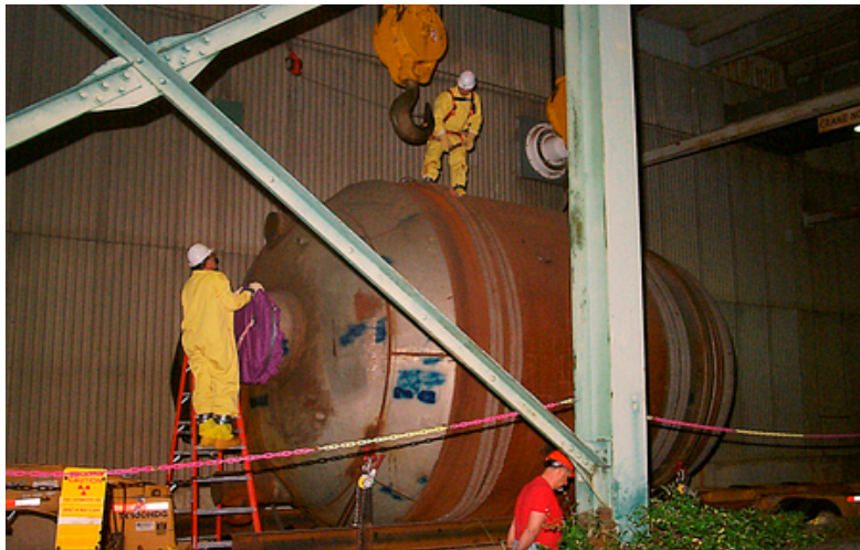
K-33 Converter Lift Complete
