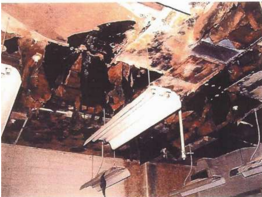
Ceiling in Bldg 2000 Room 27
