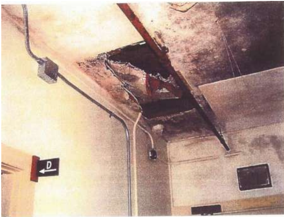
Ceiling in North Corridor at West End Bldg 2001
