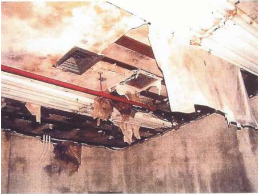
Ceiling Bldg 2001 Room D-103
