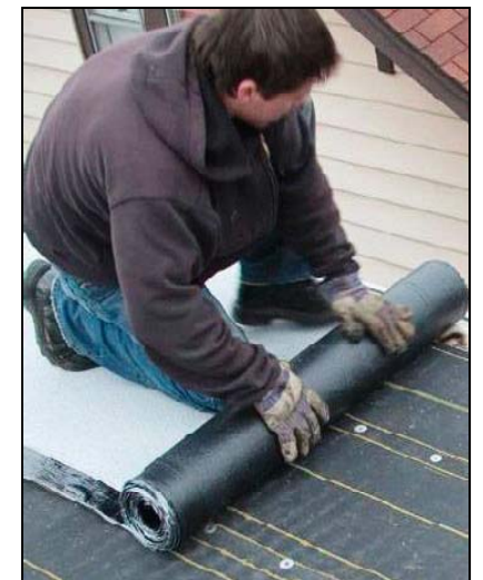
A cool coating is applied to a dark roof (top), and a cool single-ply membrane roof is unrolled (bottom). Image Source: DIY Advice
