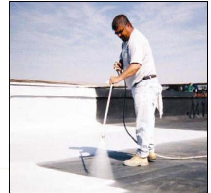
A cool coating is applied to a dark roof (top), and a cool single-ply membrane roof is unrolled (bottom). Image Source: DIY Advice
