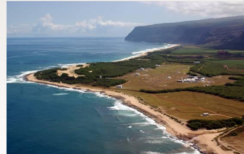
Kauai Test Facility, Hawaii
