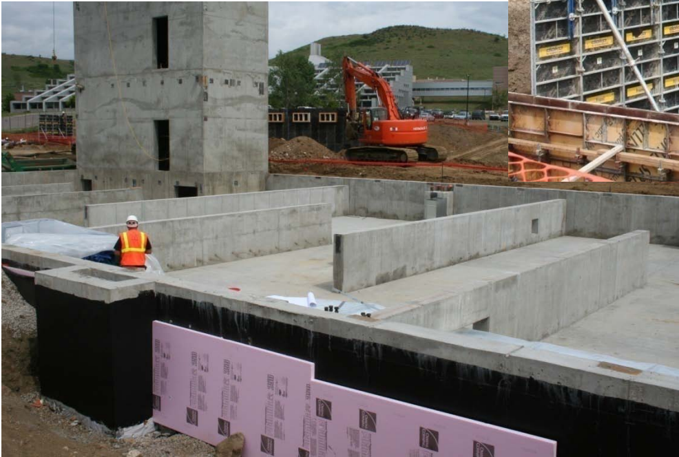
Forming Labyrinth / Stair Cores / Basement Walls – JUNE 2009
