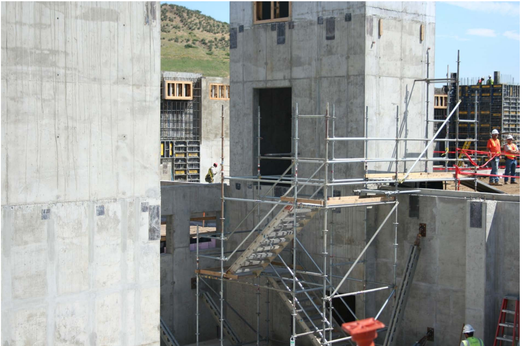
Connector Wing Ready for Grade Beams – JULY 2009
