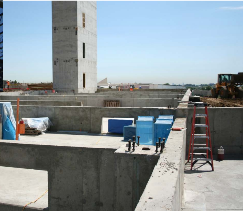
Finish Foundation Work / Backfill / Begin Structural Steel – JULY 2009
