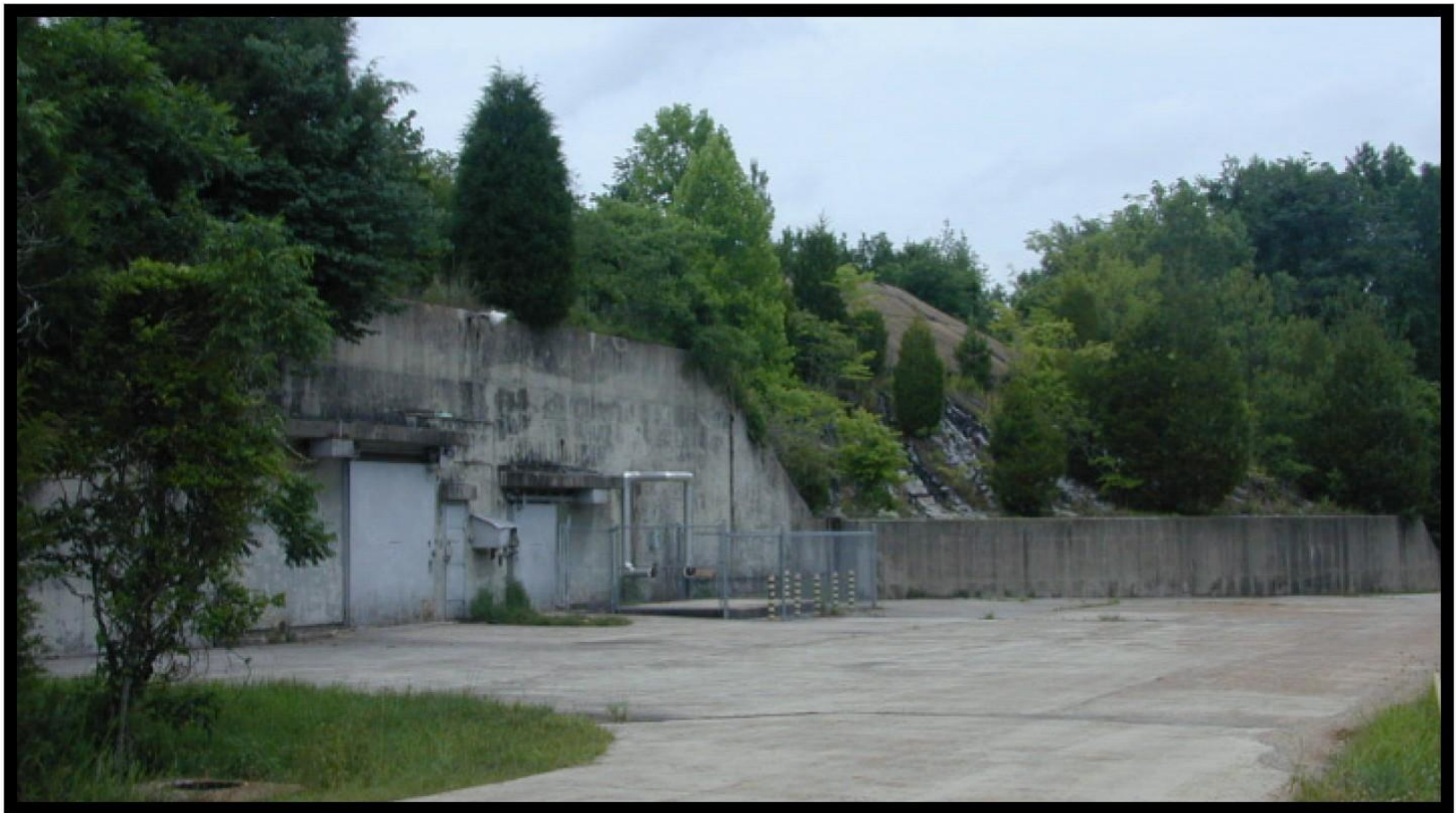
Photograph 8-25: Abandoned Gravel Gertie at the Clarksville Base. Indigenous vegetation now grows uncontrolled on the characteristic sloping roof and behind the lower retaining wall of this Cold War nuclear weapons modification plant.
